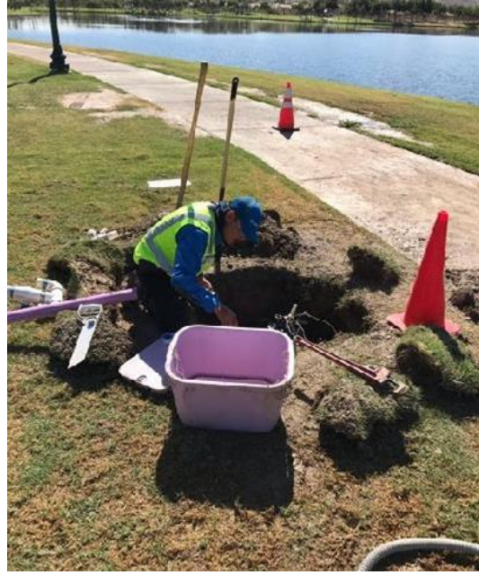
Irrigation Upgrades Continue at North Lake
