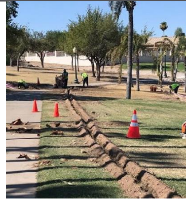
Crews Working on the Irrigation Upgrade Project
