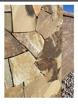
Damaged stone veneer in **Lucero** was repaired by the Exterior Maintenance Team.
