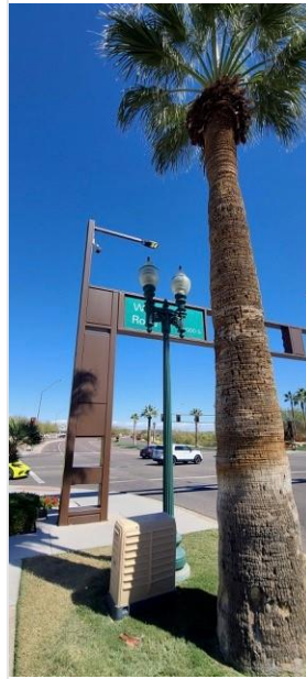
The Exterior Maintenance Team also repaired the top of an ornamental light at the corner of Estrella Parkway Elliot Road.
