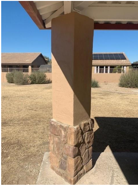
The Exterior Maintenance Team patched and painted stucco on the Ramada columns in Privada .
